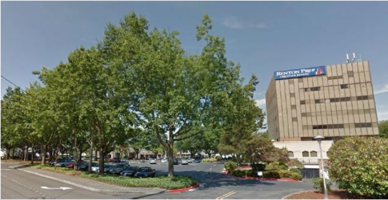
200 Mill Avenue Building and Site
